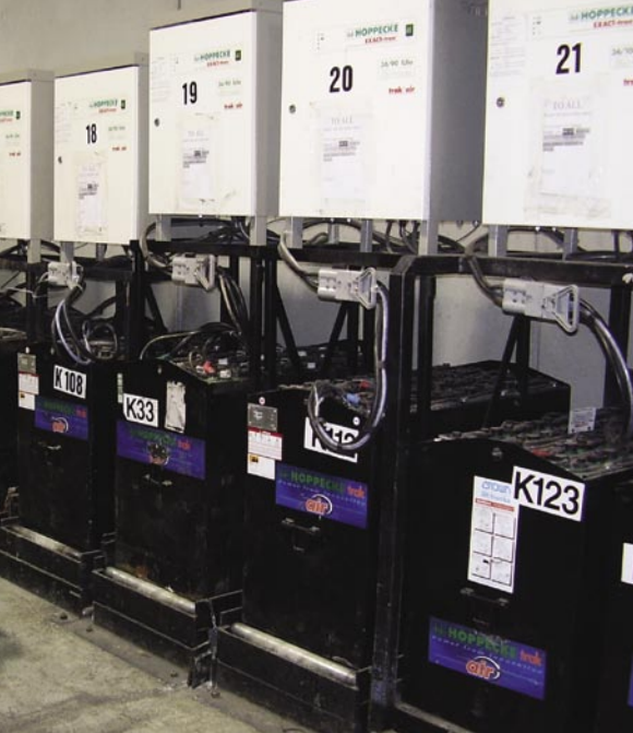
Crown supplied battery charging and watering system ensures batteries are always ready for the next shift.
