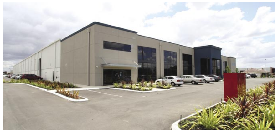
Perm-A-Pleat’s new manufacturing and distribution centre in Malaga, WA.
