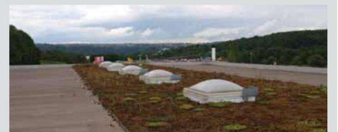
**Crown Stuttgart, Germany Branch's** roof is 1,637 square metres and is covered in vegetation. By adding an extensive green roof above the office building, Crown is able to improve the microclimate and reduce energy costs.
