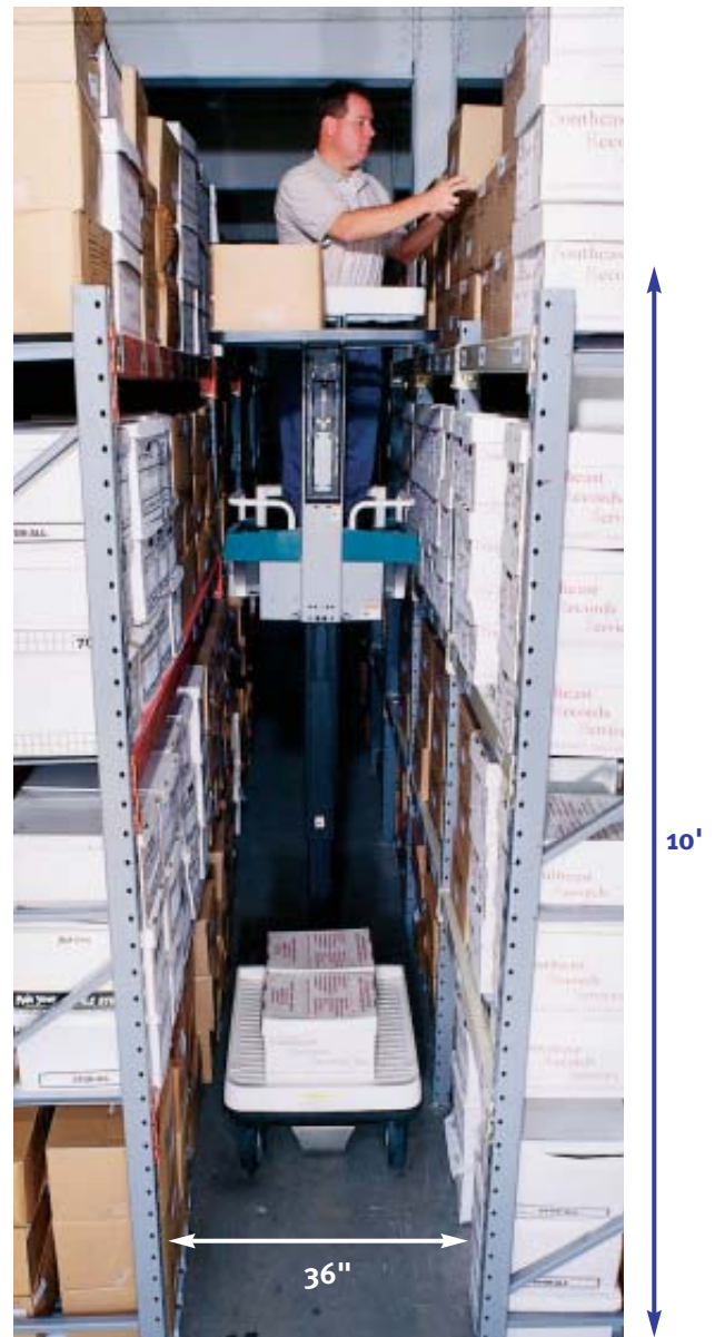
SPACE SAVINGS...SOUTHEAST RECORDS SERVICES, INC., DESIGNED THEIR GREENSBORO, NC WAREHOUSE AROUND THE WAVE. RACK UPRIGHTS ARE AT 10 FEET; AISLE WIDTHS AT 36 INCHES AND PICKING HEIGHTS REMAIN COMFORTABLE UP TO 14 FEET. COMPANY OWNERS BELIEVE THE WAVE HAS MADE A MAJOR IMPACT ON COST SAVINGS FOR THE RECORDS MANAGEMENT FIRM.
