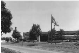
Brake Parts, Incorporated Offices & Distribution Center, McHenry, IL.
